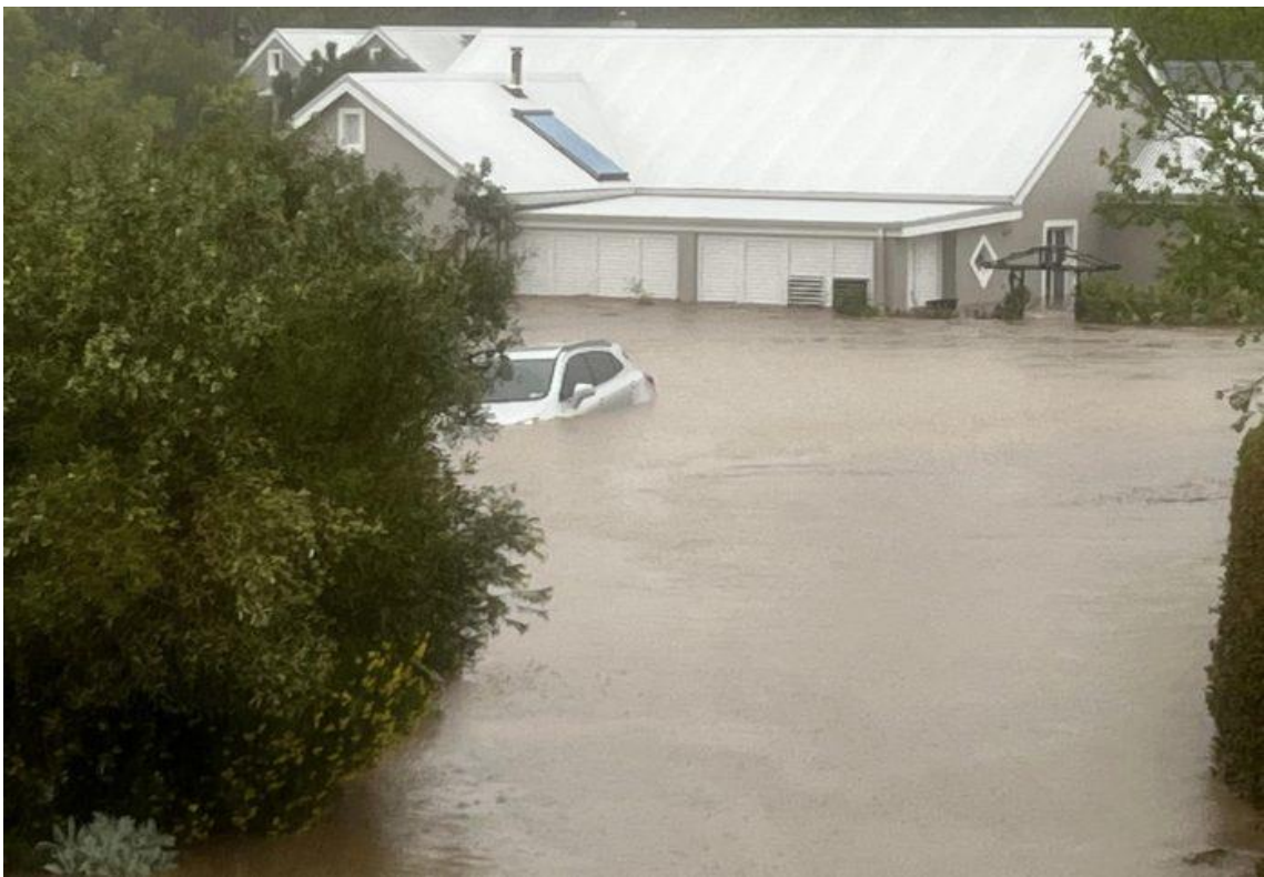
Flooding in the small Town of Stanford – 23 September, 2023
