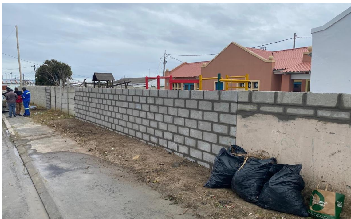
The repaired and reinforced School boundary wall as of 13 August, 2026
