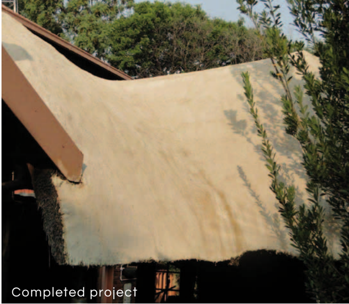
CemForce placed over thatching
